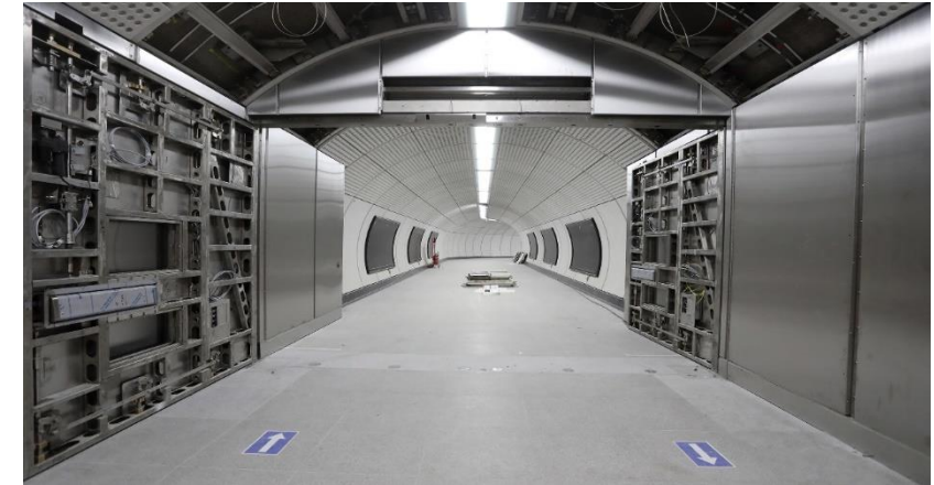
Crossrail doors installation
